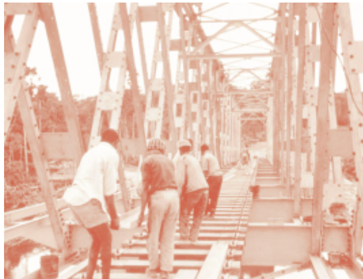
Civil constructions are important components in many Bank-assisted projects.
